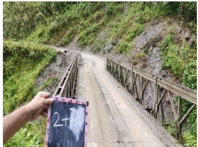
Fig 4-3: Bailey bridge at Yinkiong side
